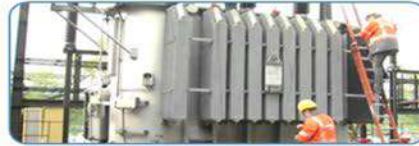
Maintenance of Transformer
